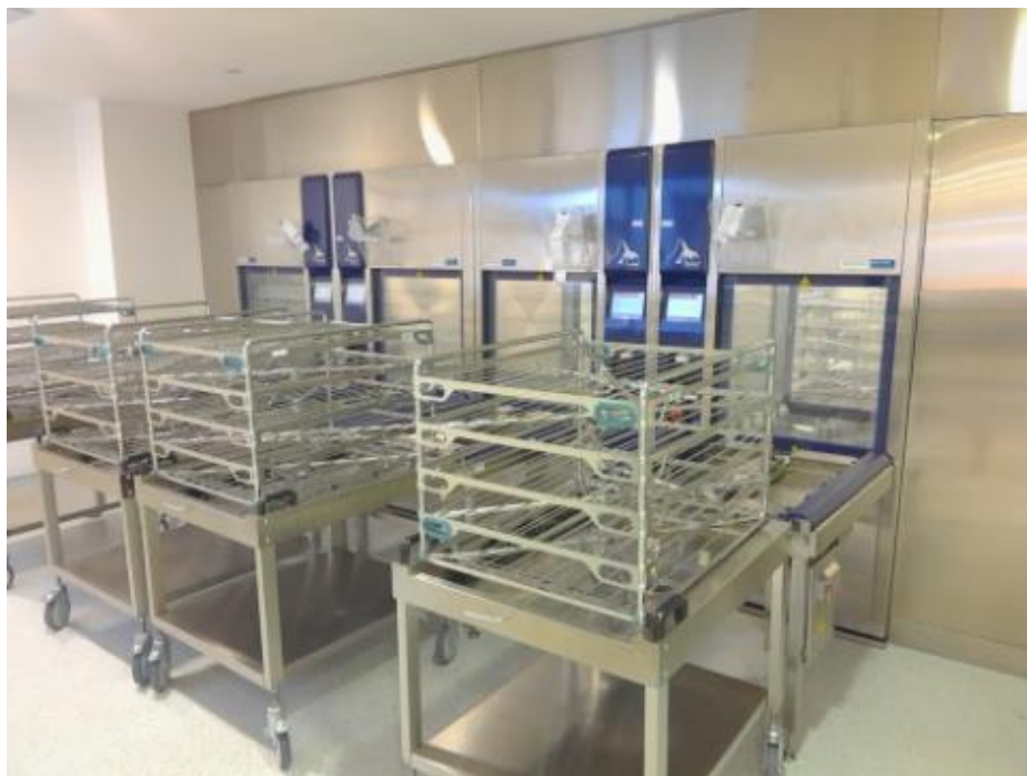
Figure 7: Sterilization with pass-through equipment leading from the packaging area to the sterile warehouse
